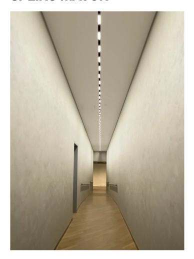
Looking into the gallery, the contrasting warm 3000K on the vertical surfaces creates an enticingly inviting atmosphere. Flexible spotlighting is semi-recessed within hand-finished plaster-in channels, a neat solution that allows the gallery to adjust the lighting to suit the current exhibition.
